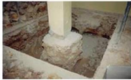
Photo 13. Excavating around the footing.
