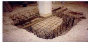
Photo 16. Completing the jacket.
