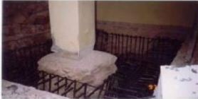
Photo 15. Installing the main steel.
