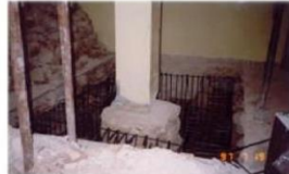
Photo 14. Hardening the surface and installing the dowels.
