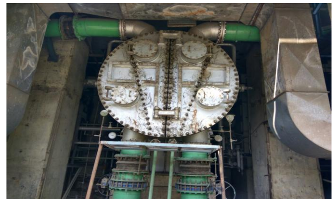
Fig:- 2.7 Surface condenser
