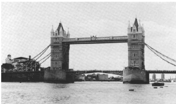
FIGURE 1.1.3 The Tower Bridge in London, completed in 1894. Note the modern beam design, made possible by the availability of steel support girders
