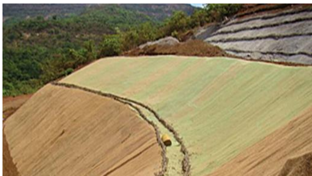
Fig3: application of jute on embankments
